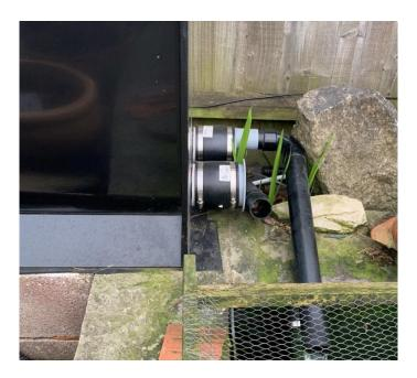
To Recap, maximum height water level should be when pumps are running is 215mm below filter top and the top of the filter should sit 370mm above pond level.
